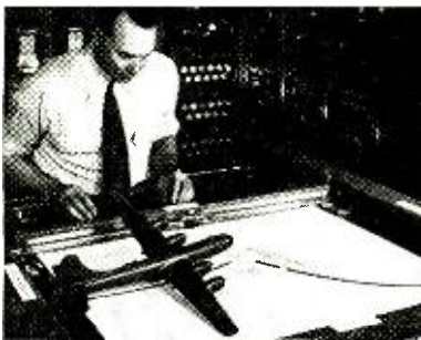
Models of guided missile and bomber about to meet on the plotting board of RCA's computer.
